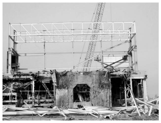
Figure 7-7 Turbine Building Demolition After Use of Explosives
