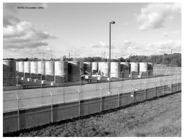
Figure 5-2 Maine Yankee ISFSI Pad and Dry Storage Casks
