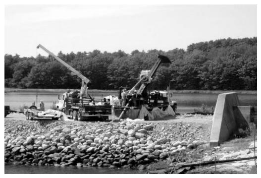
Figure 8-5 Maine Yankee Forebay Dike Core Sampling
