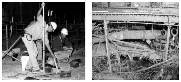
Figure 7-6 Maine Yankee Turbine Pedistal - Explosives Placement and After Detonation
